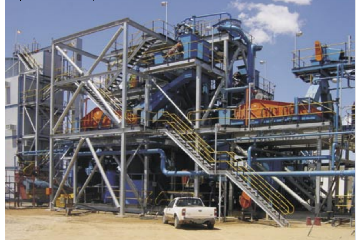
Holpan DMS and final recovery units
