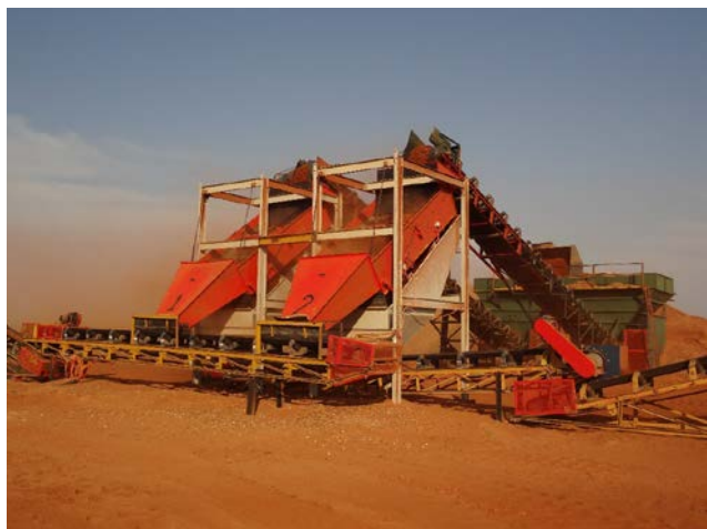
Screens (above) and containers housing the coarse- and fines streams BV plants (below) on Holsloot
